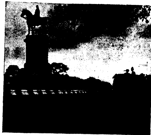
Mount Esplanade Road, Madras, laid in 1947 using 1½" Asphaltic Concrete, stands up well under heavy traffic
