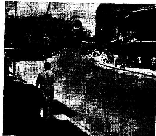
Tardeo Road, Bombay, built in 1942 with Stanvac Asphalt (3" Sheet Macadam), is still in top condition
