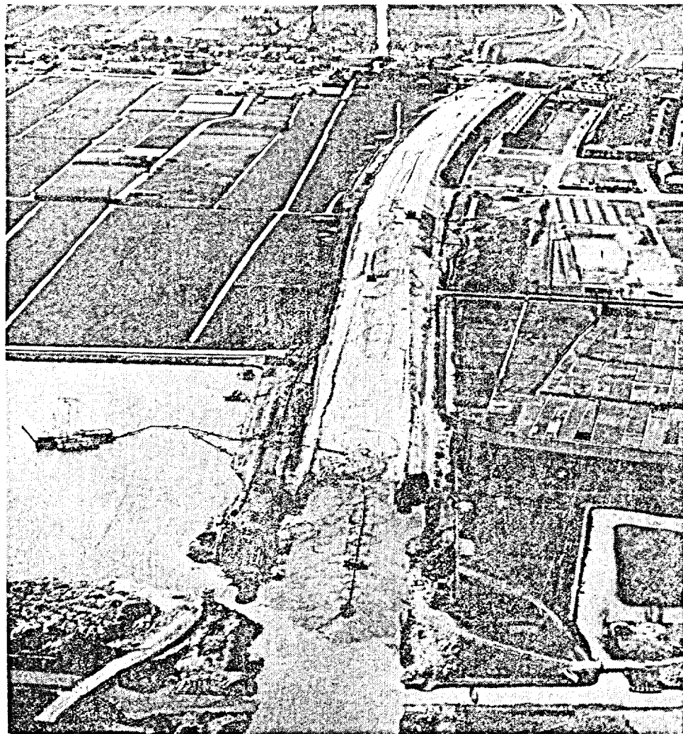
Photo 1. The road under construction. In the background: a completed section of the "earth track"; centre: work in progress on the "earth track"; in the foreground: the trench has filled with water after excavation; left: the sand pit with sand pump and delivery line for filling the trench with sand
