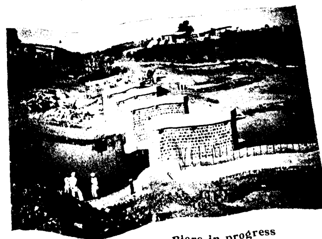
Centering of well showing kerb portion
