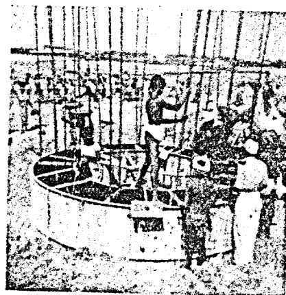
Photo 4. Concreting the well curb.
