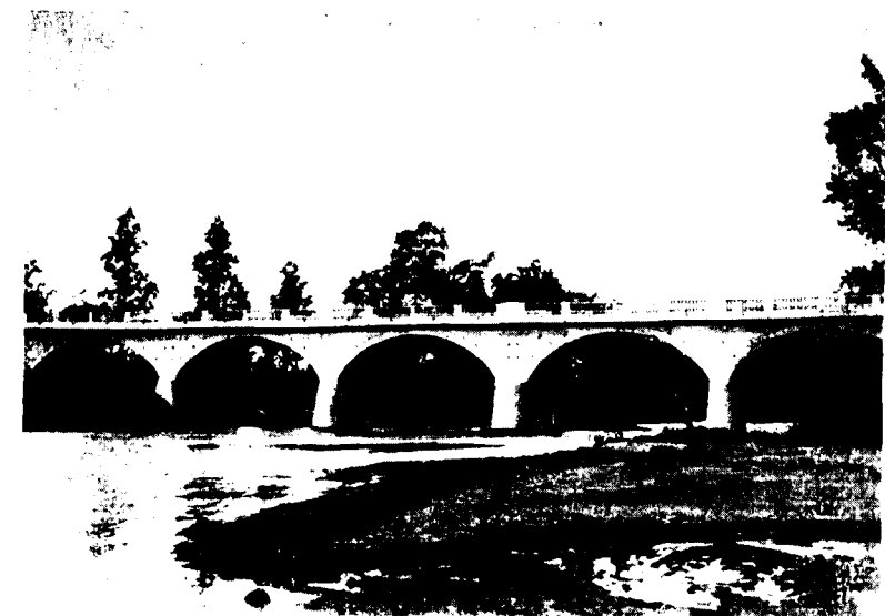
Ghogri Nallah Bridge on Jashpur-Pathalgaon Road, 5 spans of 38 ft each.
