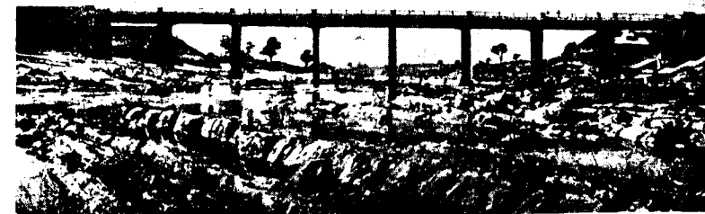
Kele Bridge, 8 spans of 40 ft each
