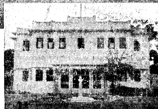
Administrative block of the Rural Health Unit and Training Centre, Singur.
