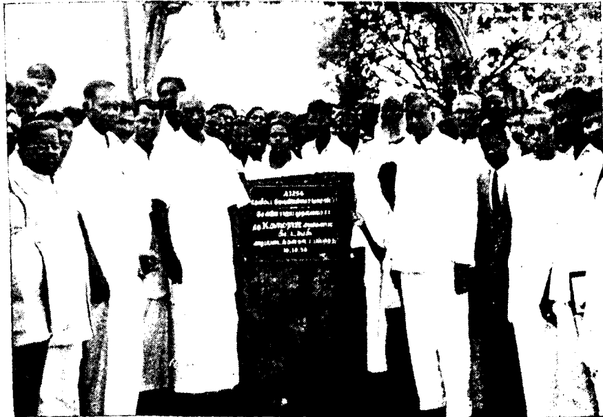
Sri K. Kamaraj, Chief Minister, laid the foundation stone for the construction of a godown by the Theni Co-operative Sale Society at Chinnamanur in Madurai District on the 10th October, 1956.
