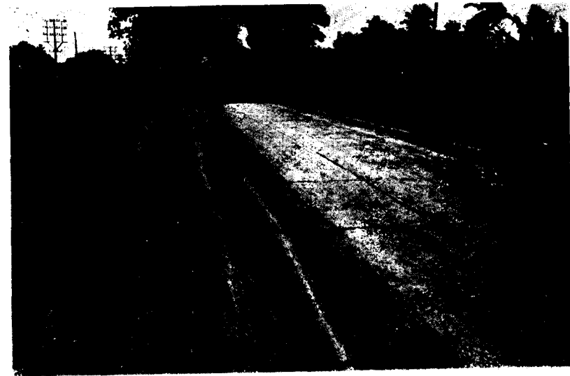
Photo 1. Great Western Trunk Road at mile 4/5 between Madras and Poonamalle.
