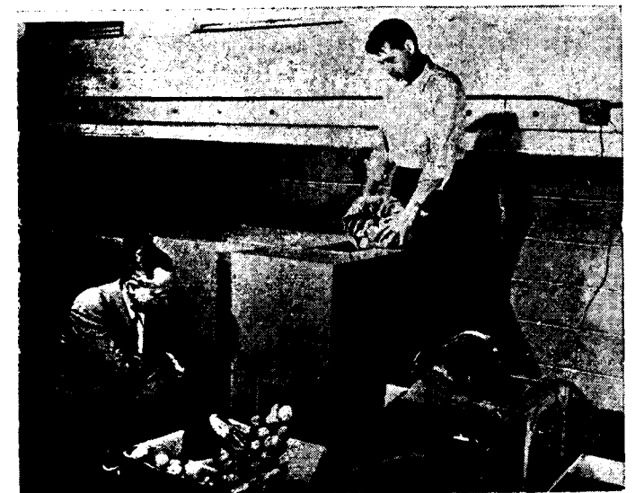
Potatoes properly exposed to radiation do not sprout, wither or spoil for two years. This portable atomic-processing unit can be mounted on a truck and moved into a field, where it can quickly "preserve" an entire potato crop.
