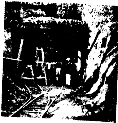
Photo 4. The beginning of No. 2 tunnel draft face
