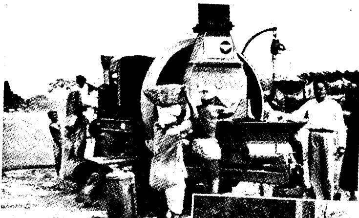
Illustrations show a Parker 'SPOT-MIX' plant working for the Patna Improvement Trust.
