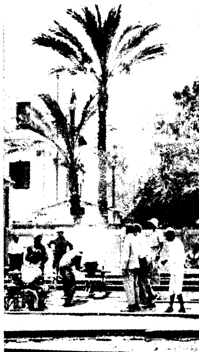
Welding in tracks.
