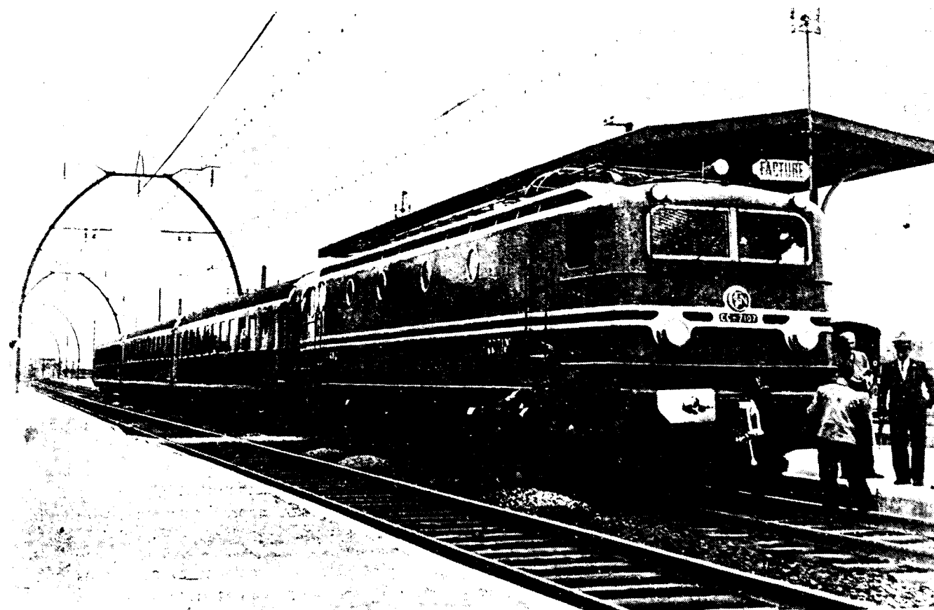
This CC 7107—1500 V, 107 f, 5000 HP. locomotive has reached on March 28, 1955 the speed of 206 mph.
