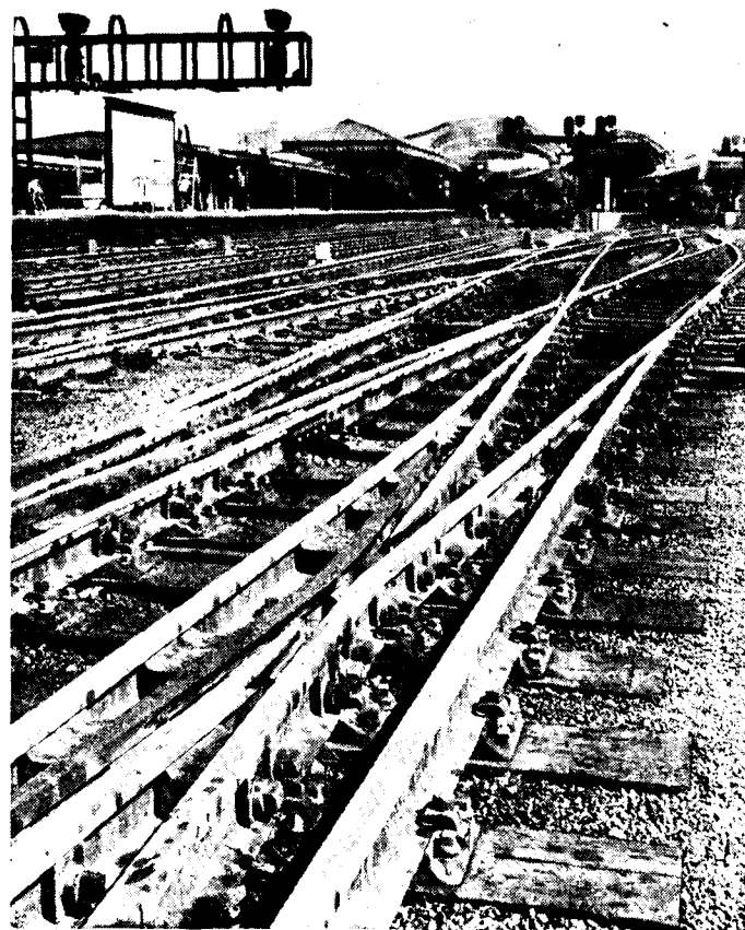
Fig. 3. Rail Clips at an important Junction of British Railways system. (Photo: Courtesy of British Railways)
