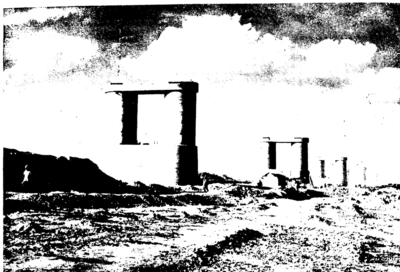
Main Piers 15 to 11 completed upto bed stone level. Top of cap at R.L. + 172. Base of 15 ft. dia. reinforced concrete cylinders at R.L. + 143.
