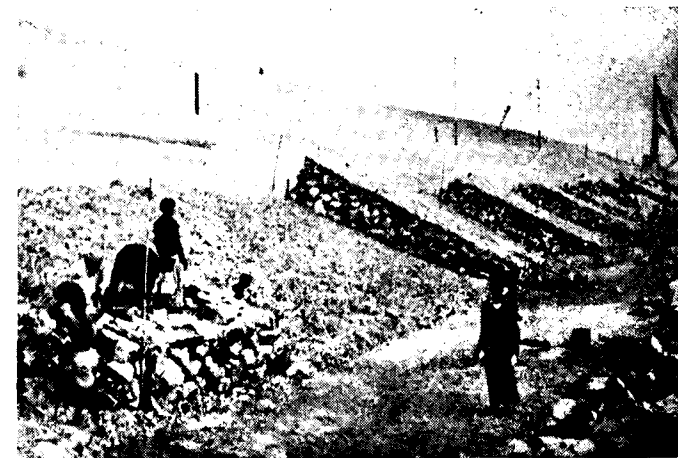
View of Guide Bank—Protection of Front Side Slopes with 9" quarry refuse and 3 1/2 ft. thick boulders hand-packed.
