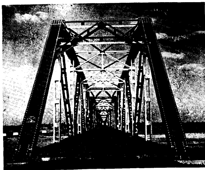
End view of the new bridge at Sevalia which was opened for traffic from 28th September 1954. This bridge was built at a cost of half a crore of rupees.
