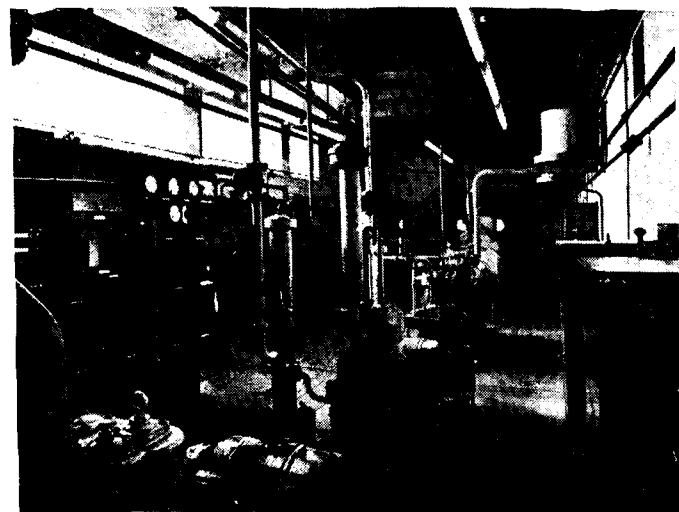
Standby diesel generator set, air compressors, and switchboards for power supplies to the signalling.
