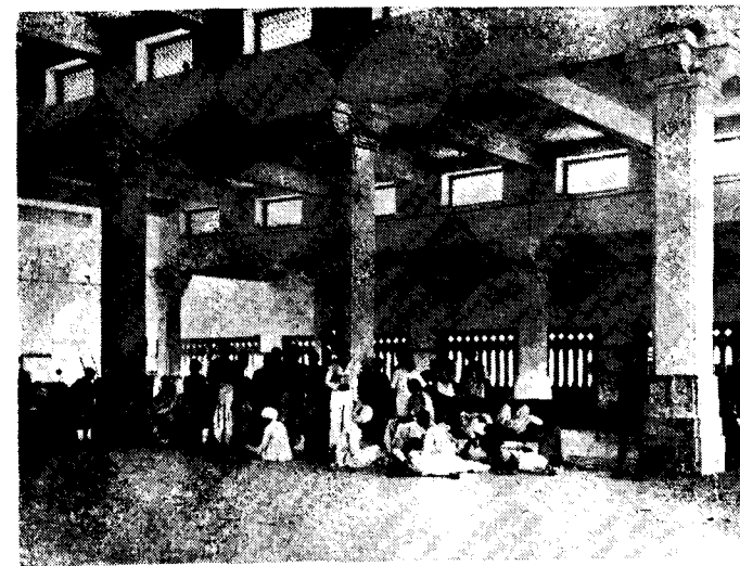
Third class waiting hall at the newly built Mehsana Station.
