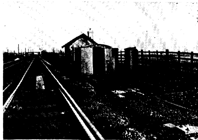
Point layout showing Point Machine and Asbestos Hut Housing the Battery Point Motor rates 30 volts 5.5 amperes maximum operating time 6.0 seconds.
