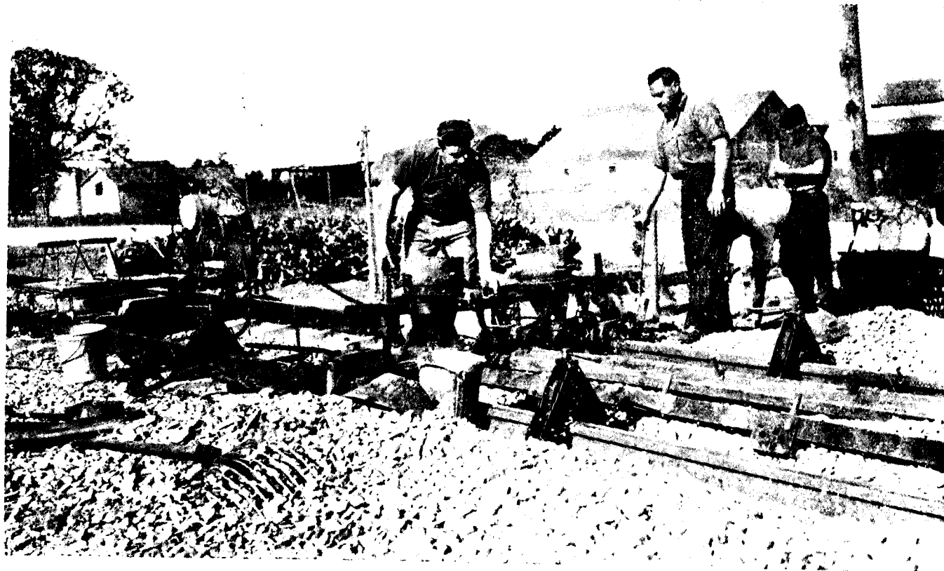
Fig. 5. Welding of rails.
