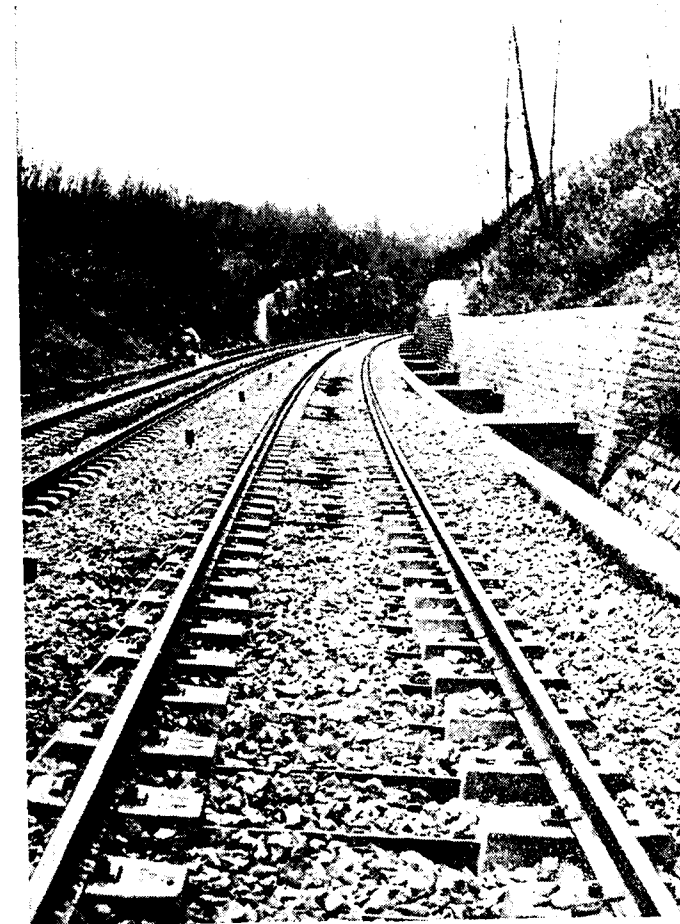
Long rails (900 m) on Vagneux concrete ties type 1954 with
