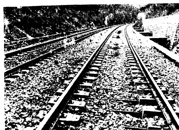
Long rails (900 m) on Vagneux concrete ties Type 1934 with "bolt-tie bolt" Vagneux, spring clip "RN" and grooved rubber-tie pads
