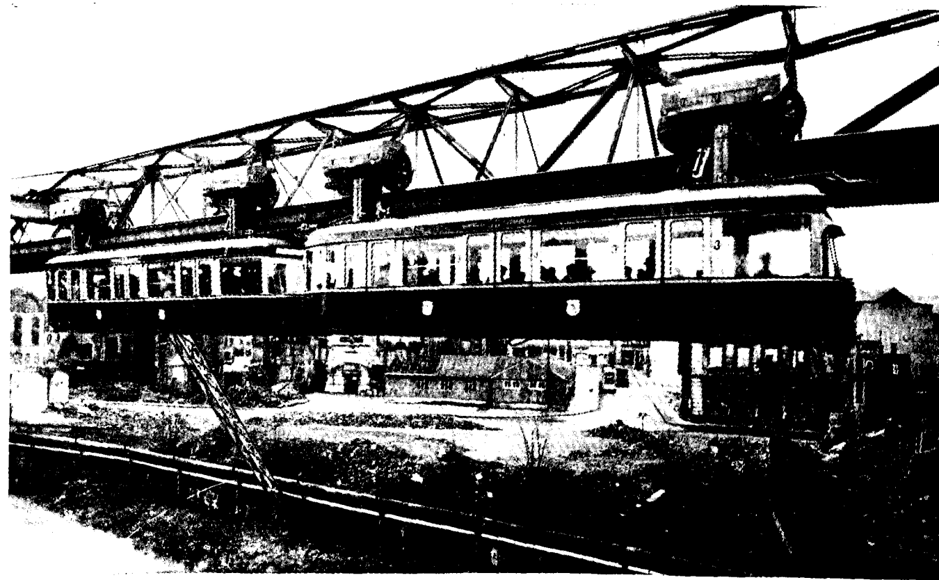
Fig. 3. Hanging train over the River.
