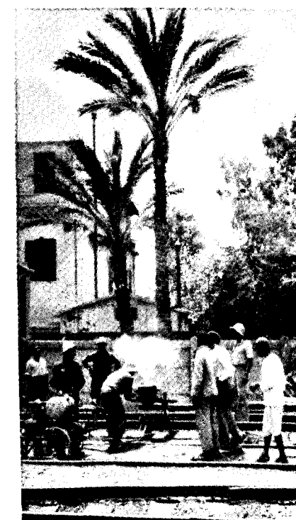
Welding in tracks.
