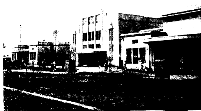
The new Mehsana Station, which was opened in July 1954.
