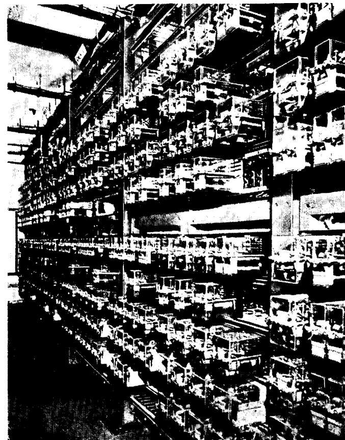
Rack of plug in signal relays.
