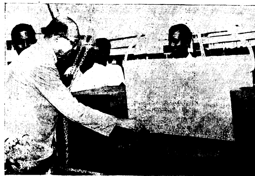
Shri D. N. Mitra laying the foundation stone of the Students' Hall of the School of Printing Technology, Calcutta.
