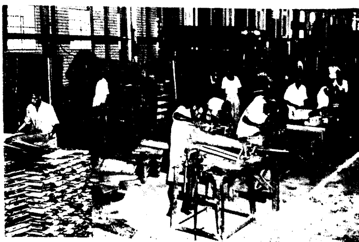
Fabricating of sheet metal components at Ashok Leyland's at Ennore
