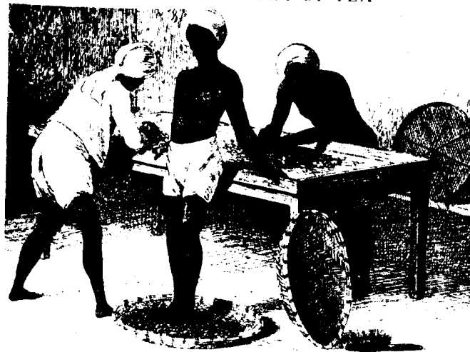
1. Old method of rolling leaf by manipulation with the hands and feet. (By courtesy of Davidson and Co. Ltd, Belfast.)
