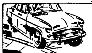
(2) Driven repeatedly over kerb with deliberate violence. No loss of air despite three 3" nails in the tyre.
