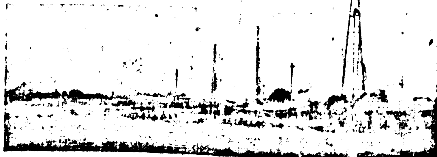
The drill at work. Drilling a hole of 26 to 27 inches in a depth of 400 feet is no easy matter.
