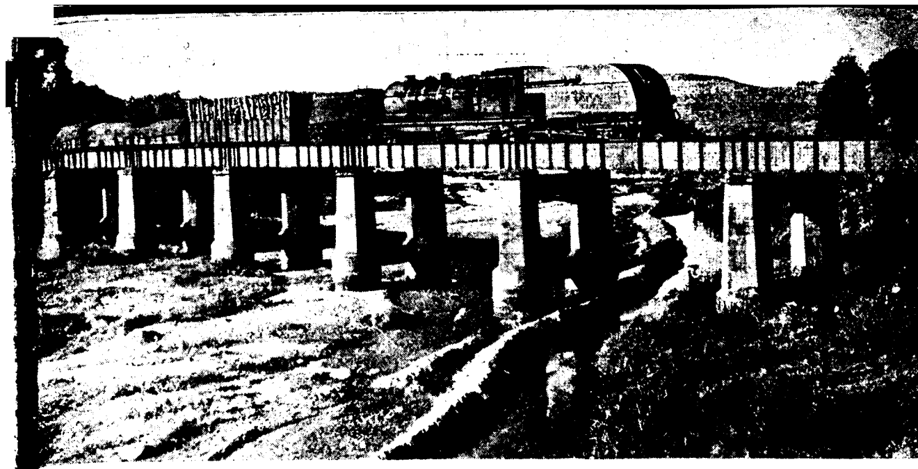
A powerful GEA type Beyer-Garratt steam locomotive, heading a heavy goods train on the Cape Town-Port Elizabeth route
