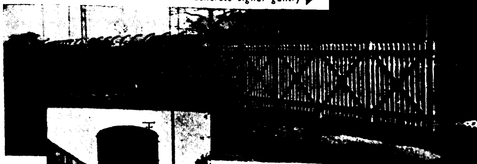
Precast concrete fencing in railway yard
