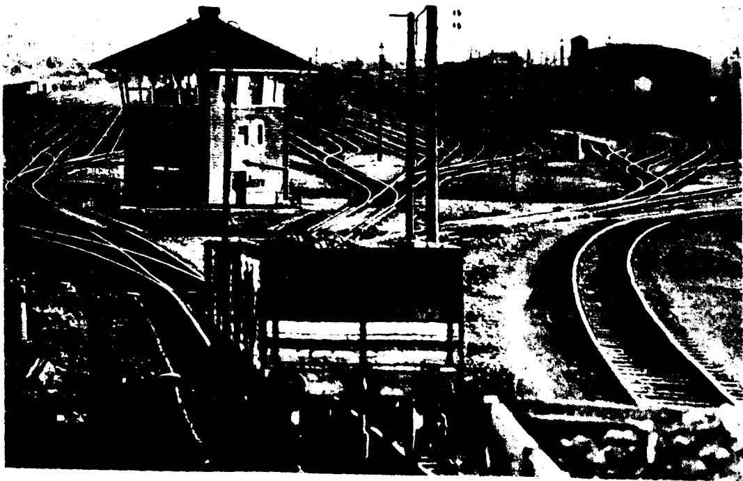
A general view of the Whitemoor Marshalling Yard in England described in this article
