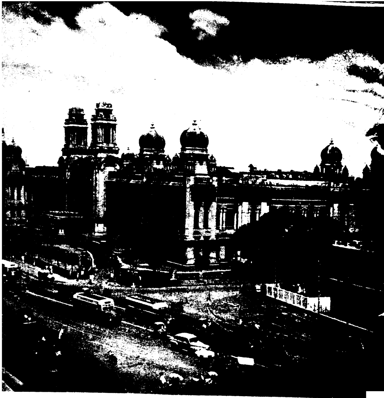
Southern Railway Headquarters Offices, Madras
