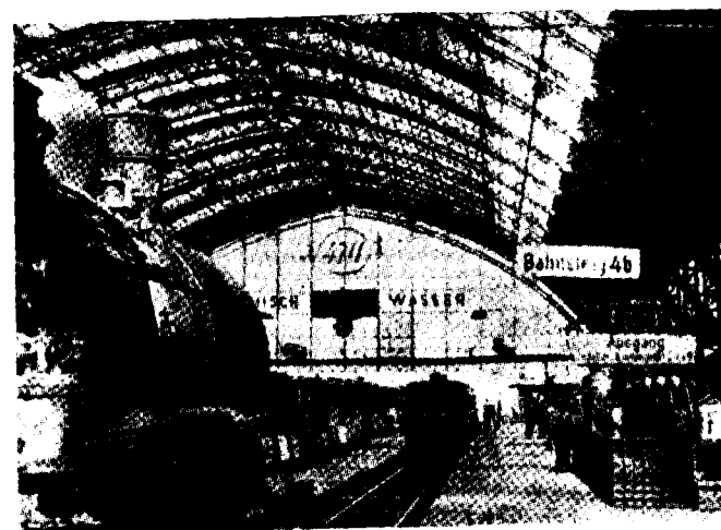
Cologne Central Station interior. New signalling permits three trains standing on each platform line at the same time
