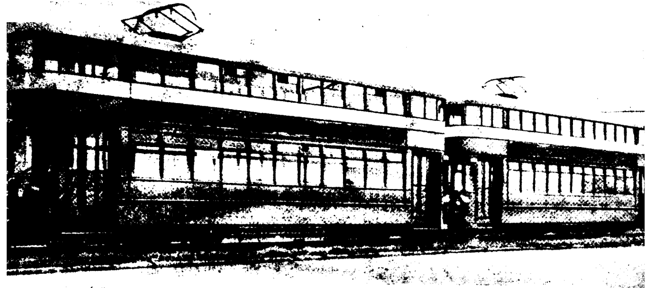
A modern two-car, double-decker train on the electrified Swansea and Mumbles Railway, seating 212 passengers
