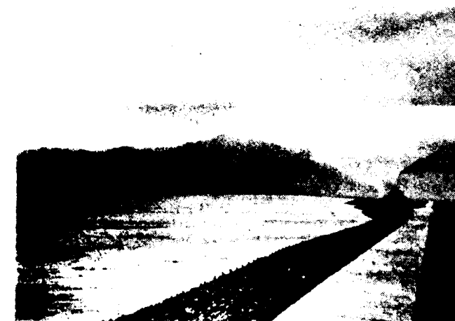
Entrance to the dam—the Kotagiri mountain can be seen in the background
