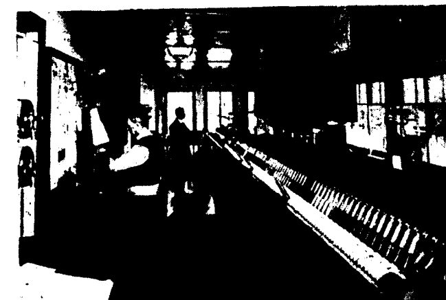
Auckland Signal Box of the New Zealand Railways with 128-lever electro-pneumatic inter-locking machine
