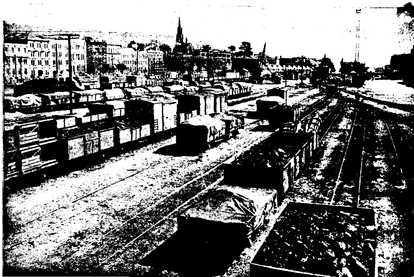
The commodious city goods yard of the New Zealand Railways at Dunedin
