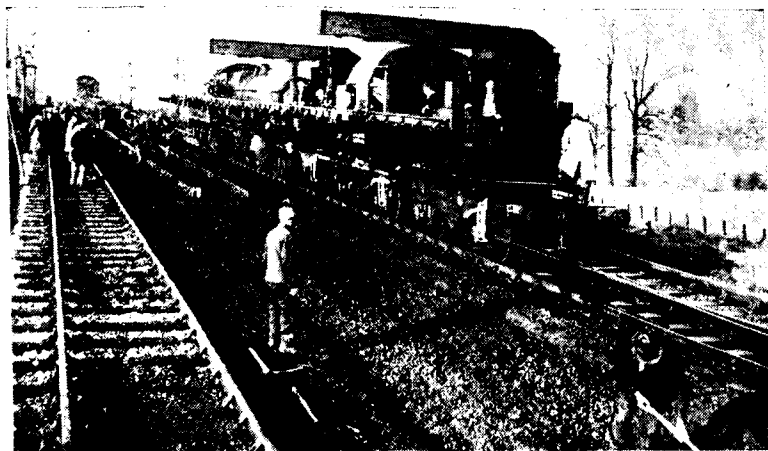
Mechanical laying of pre-assembled 4' 8½" gauge track on the Western Region of British Railways
