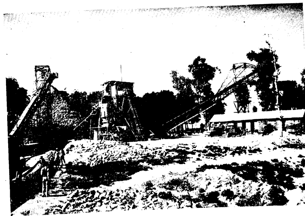
President Rajendra Prasad laid the foundation stone of the Ganga Bridge on 25th February, 1956. Above : 43 feet high caisson weighing 300 tons laid for pier No. 2. Sinking is in progress. Below : Crushing plant with a capacity of 90 tons per hour for manufacturing aggregate for the foundations of the Ganga Bridge
