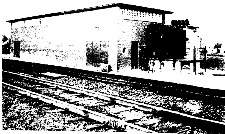
Typical unattended sub-station on the Dutch electric routes near Maastricht
