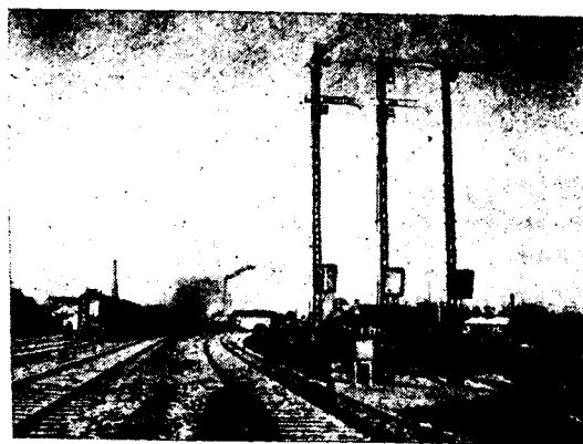
Typical modern metal lattice signal equipment on the Danish State Railways
