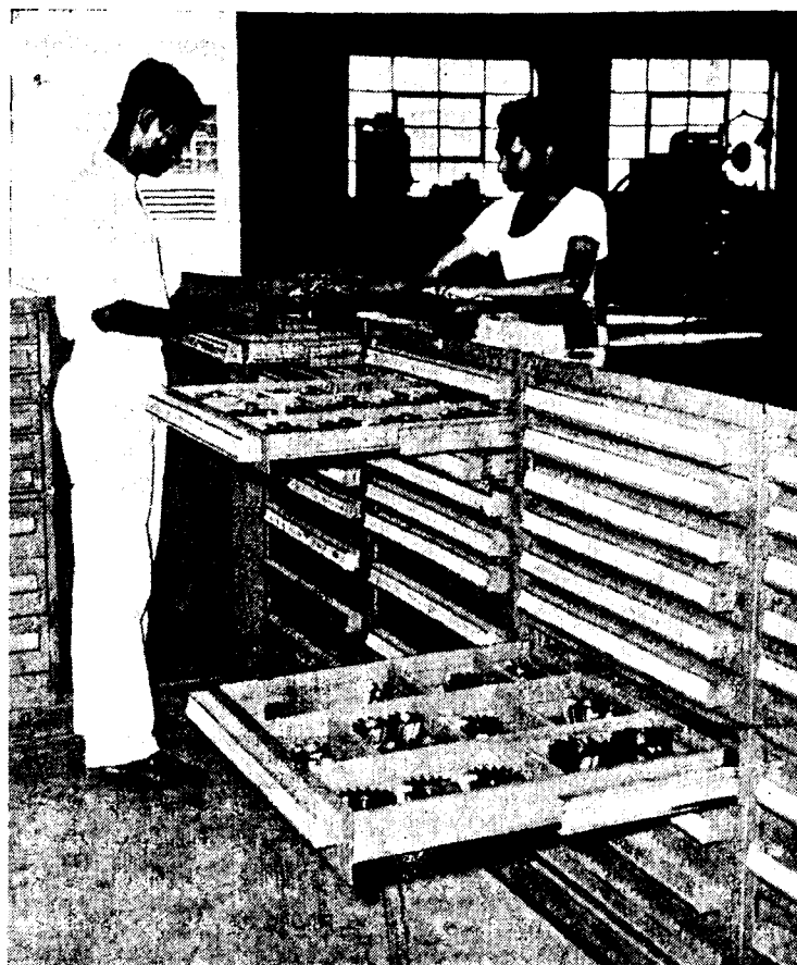
Tool cribs—(The drawers slide on telescopic ball-bearings)
