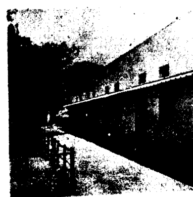
V. M. High School Building at Bodi (Madurai Dt.)
