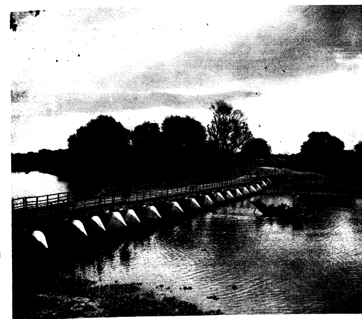
The pontoon bridge on the Barhampur-Jalangi State highway
