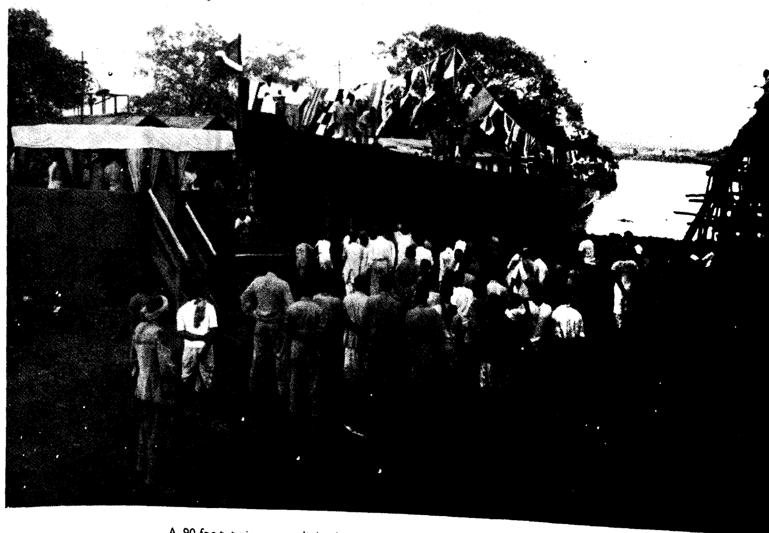
A 90-foot twin-screw, light-draught towing launch about to enter the water
