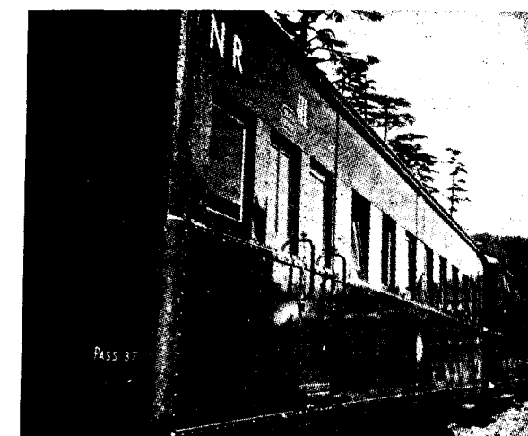
A narrow gauge aluminium panelled coach
