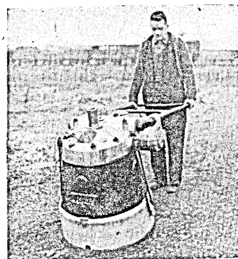
Big Problems - The Johnson Frog Rammer is suitable for Earth Dams, Bunds, Canal Work, Railway Embankment, etc.
