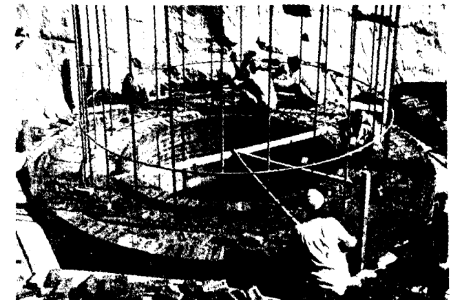
Masonry for wells in progress.
