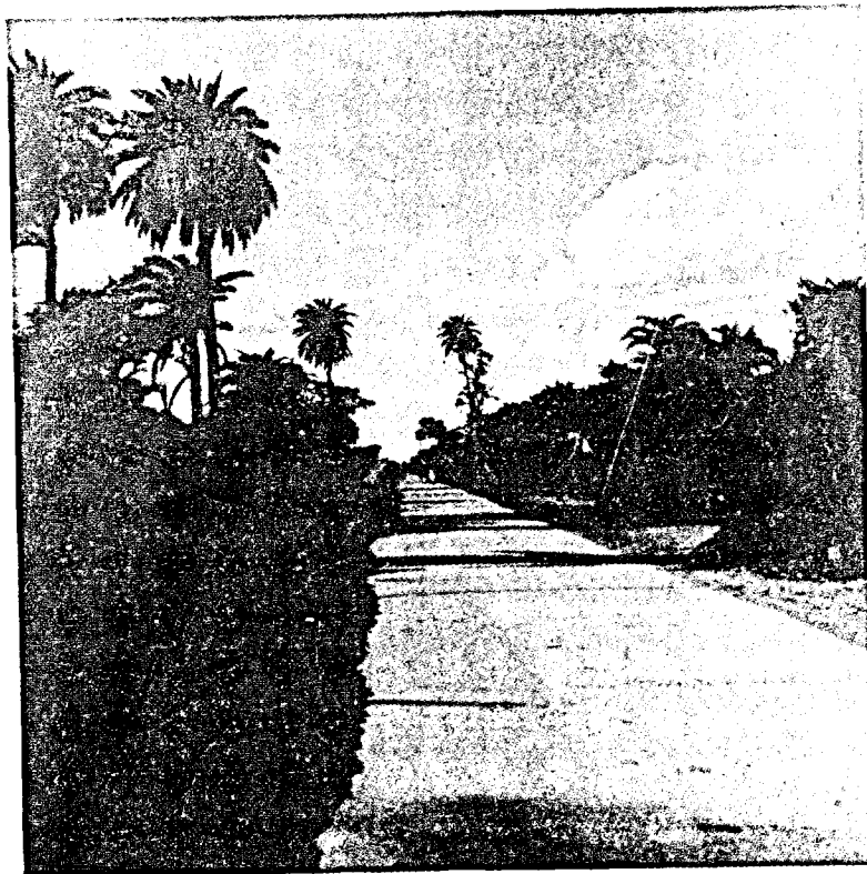
CONCRETE SURFACING IN AGRA-BOMBAY ROAD— MADHYA PRADESH
