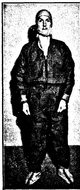
FIG. 5.—Original immersion suit made of fabric which allows the passage of water vapour—i.e., perspiration—but is waterproof. It was designed to keep a man's clothing dry after ditching before boarding his dinghy or being picked up. (Air Ministry Crown copyright.)
