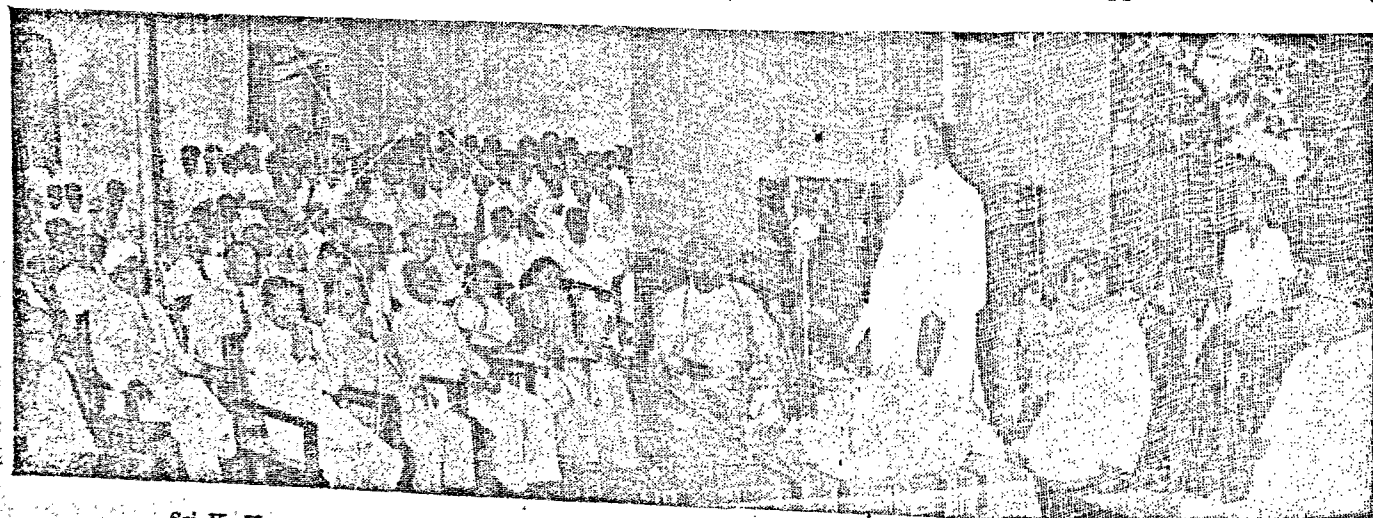
Sri K. Kamarsj, Chief Minister, addressing the function held in connection with the opening of the new administration building of the Government Transport.
