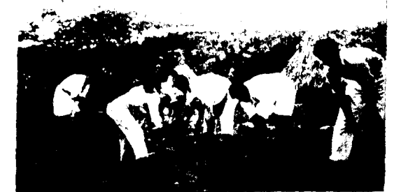
Levelling a road. Rural Service League Annual work camp at Meppedu Village
