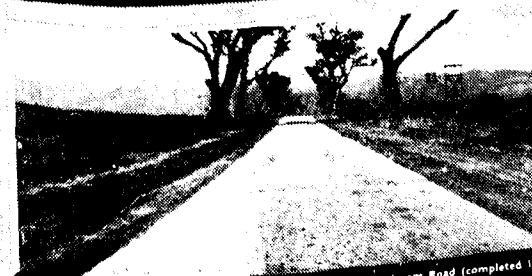
Coimbatore-Mettupalayam Road (completed 1948)
