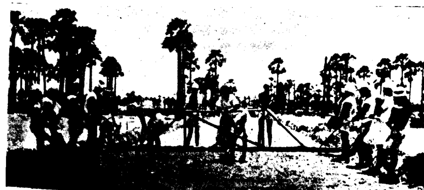
Photo 7. Spreading and levelling to camber
