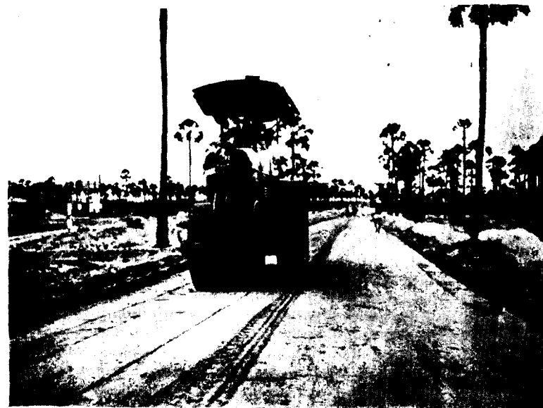
Photo 9. Final compaction with smooth-wheeled power roller
