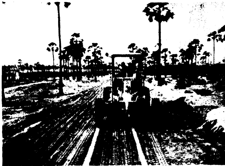
Photo 8. Initial rolling with pneumatic tyres
