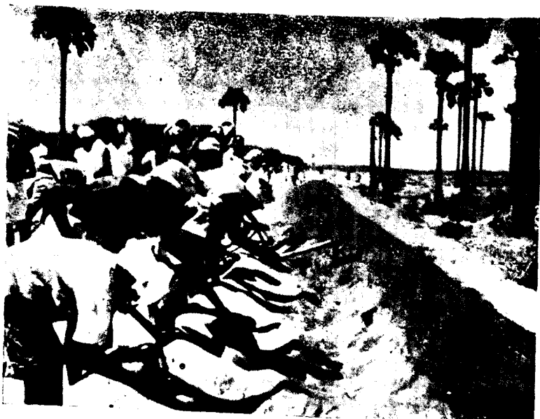
Photo 3. Dry mixing of sand and clay
