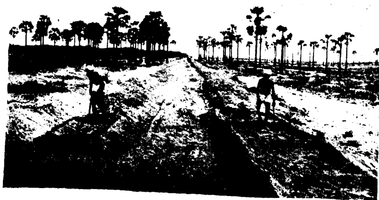
Photo 4. Forming bays for watering
