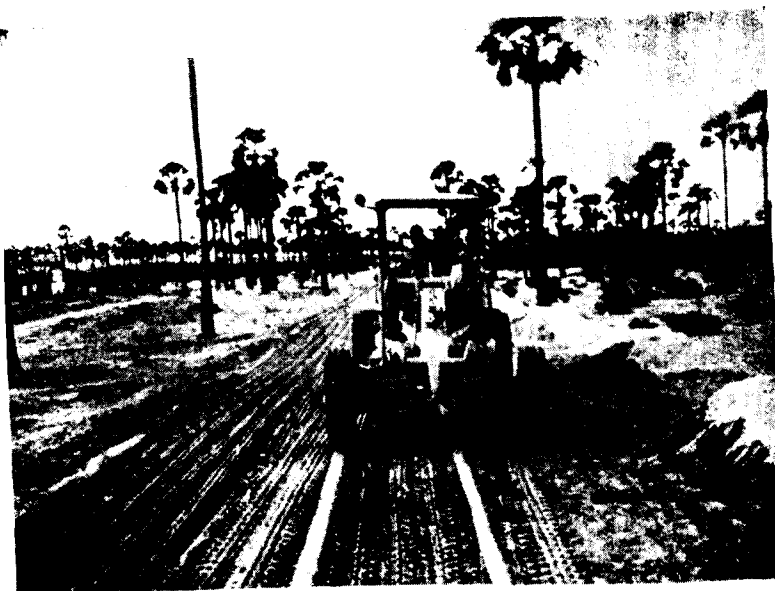
Photo 8. Initial rolling with pneumatic tyres
