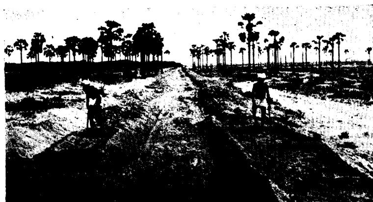
Photo 4. Forming bays for watering
