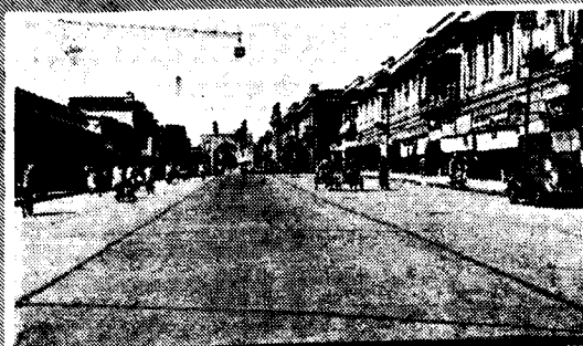
Char Minar Road, Hyderabad (completed 1929)
