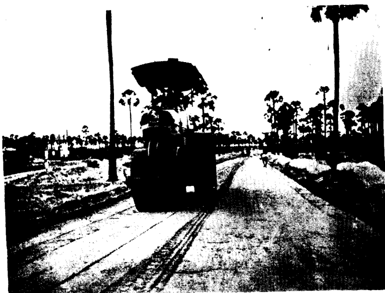
Photo 9. Final compaction with smooth-wheeled power roller
