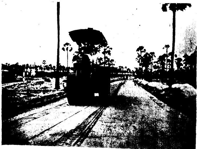
Photo 9. Final compaction with smooth-wheeled power roller
