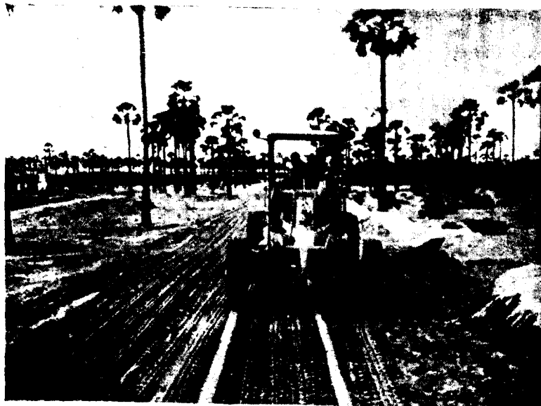
Photo 8. Initial rolling with pneumatic tyres
