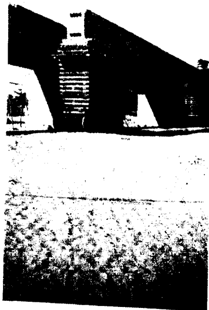
Photo 19. A beam on the move on the river bed
