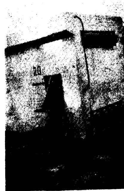
Photo 13. Fixing of the wires after tensioning by driving in the wedge
