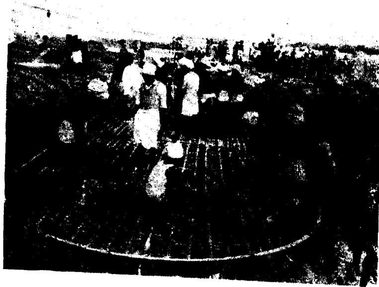
Photo 7. Concreting the capping slab
