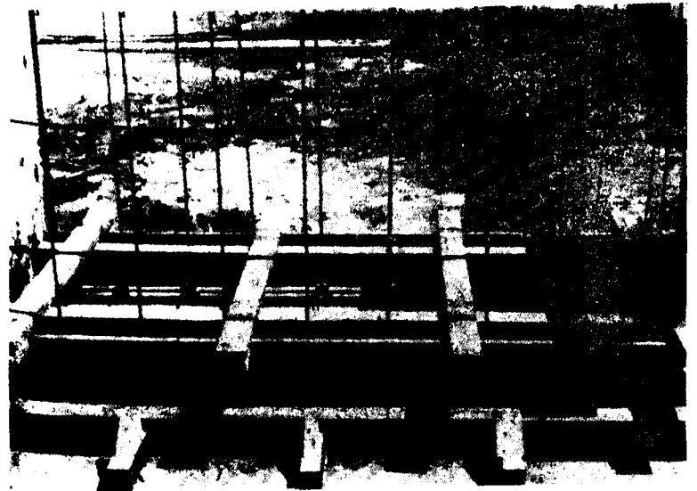
Photo 9. Shuttering for the soffit slab
