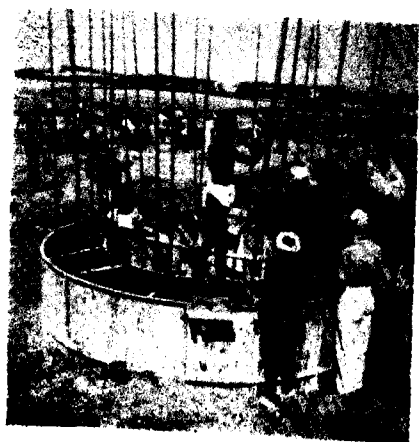
Photo 4. Concreting the well curb
