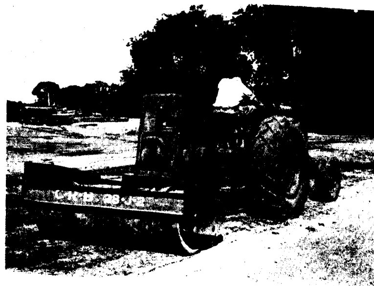
Photo 2. Vibrating Roller at work
