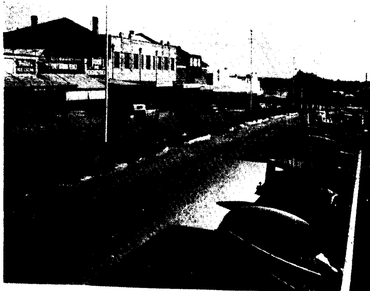
Photo 10. Median strip in a main street—Leeton
