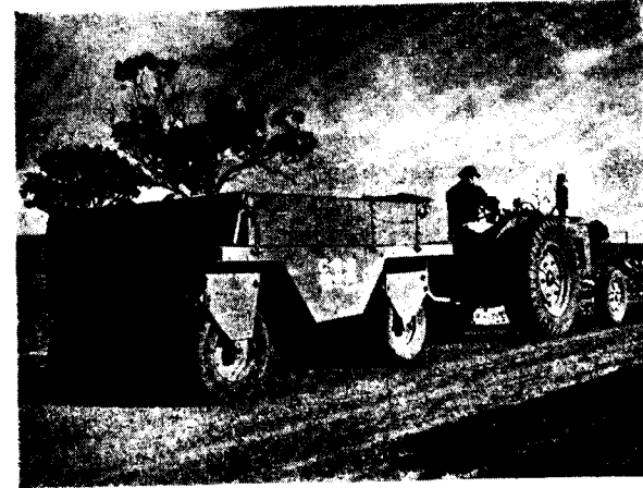
Photo 6. Pneumatic tyred roller at work
