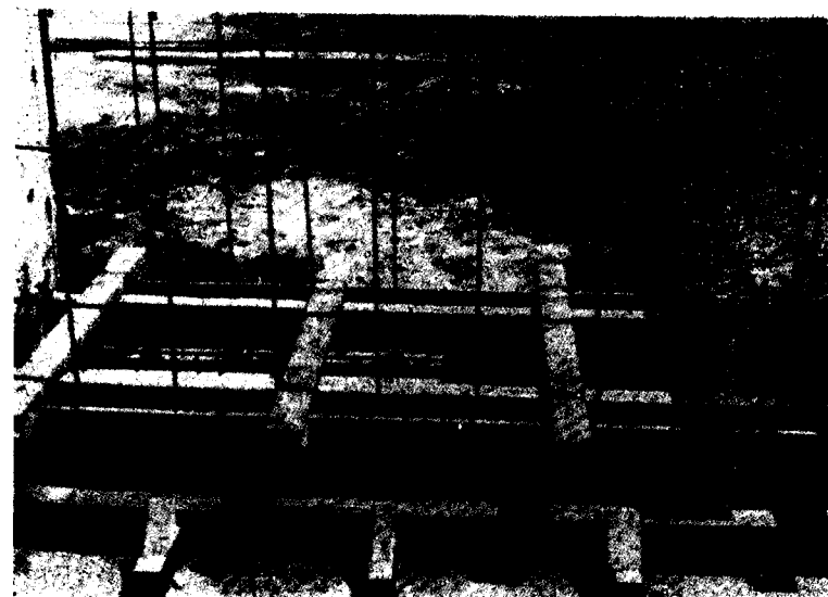
Photo 9. Shuttering for the soffit slab
