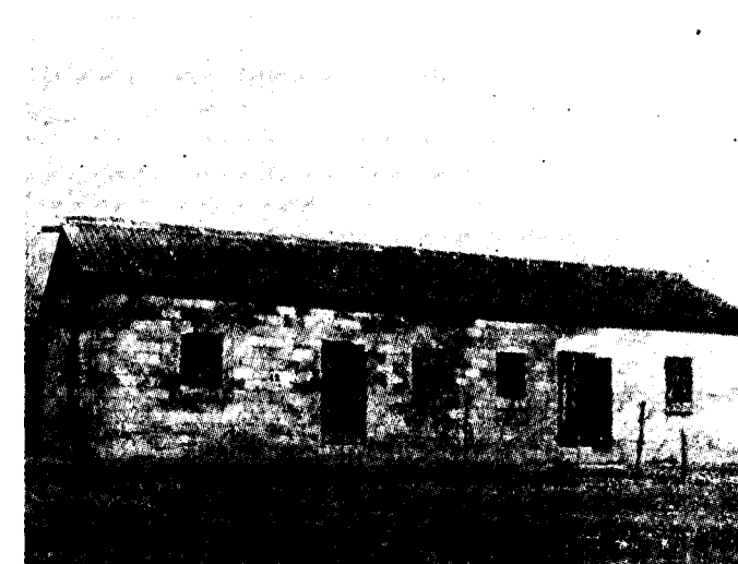
Two roomed Hollow Concrete Block Quarters.
