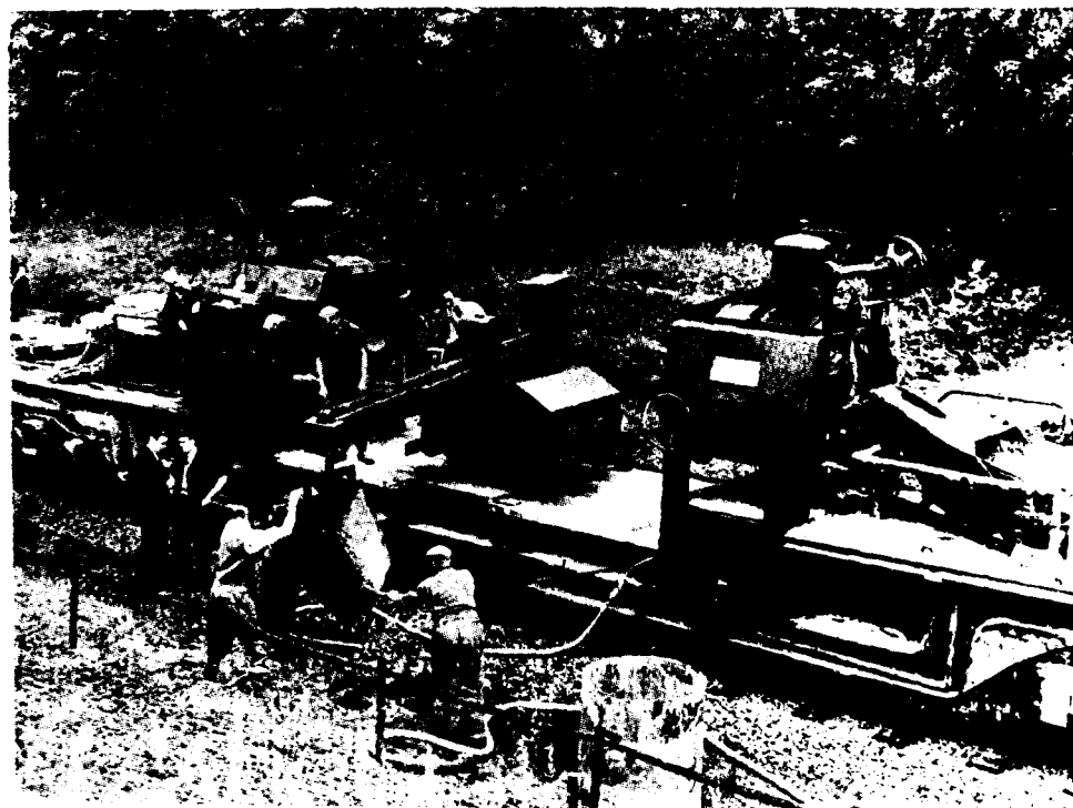
Mixing and placing unit pouring concrete round steel core former.
