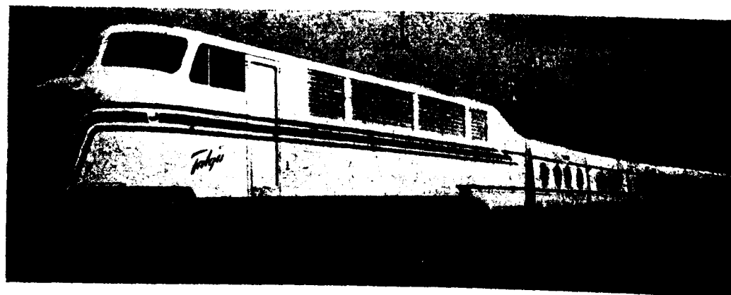
The demonstration A.C.F.-Talga train consisting of a locomotive, a baggage unit and a coach of five units. In this dramatic development all-aluminium construction has resulted in the coaches being only one-fourth the weight of conventional steel stock. (Patentes Talga and American Car and Foundry Company).
