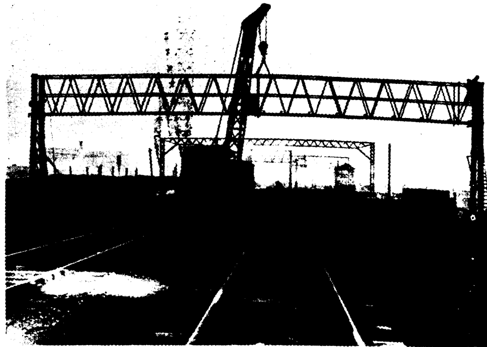
Erecting the bridge of a multi-track anchor structure—London to Shenfield Electrification.
