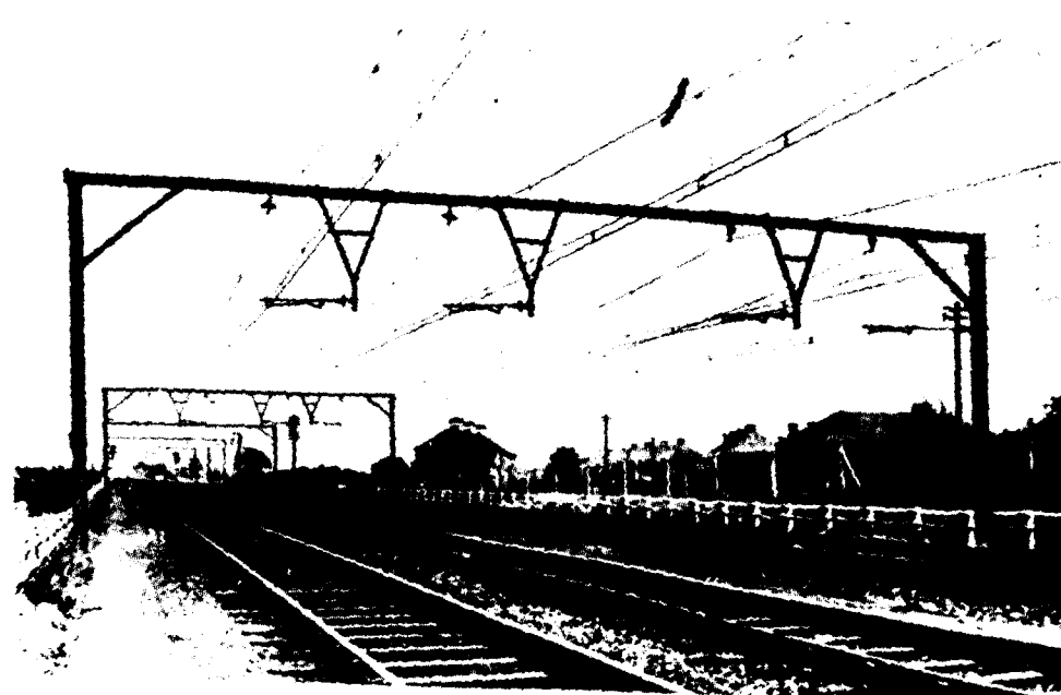
Four-track, broad flange beam portal structure. Showing a method of "registering" (i. e. locating) the contact wire and auxiliary catenary wire over each track. The wires are arranged in compound catenary form.—London to Shenfield Electrification.
