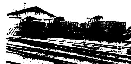
Sulzer Diesel-electric shunting locomotive of 735 H.P. owned by the Societe Nationale des Chemins de Fer Francais (supplied in 1938). Their experience with these locomotives led the S.N.C.F. to order numbers of other shunting locomotives with Sulzer Diesel engines.
