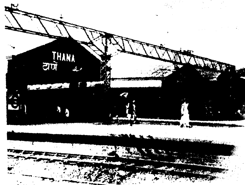
Lattice-type supporting structure at Thana, Central Railway, India. Note the bird guards over the insulators to prevent accidental earthing of the overhead equipment.
