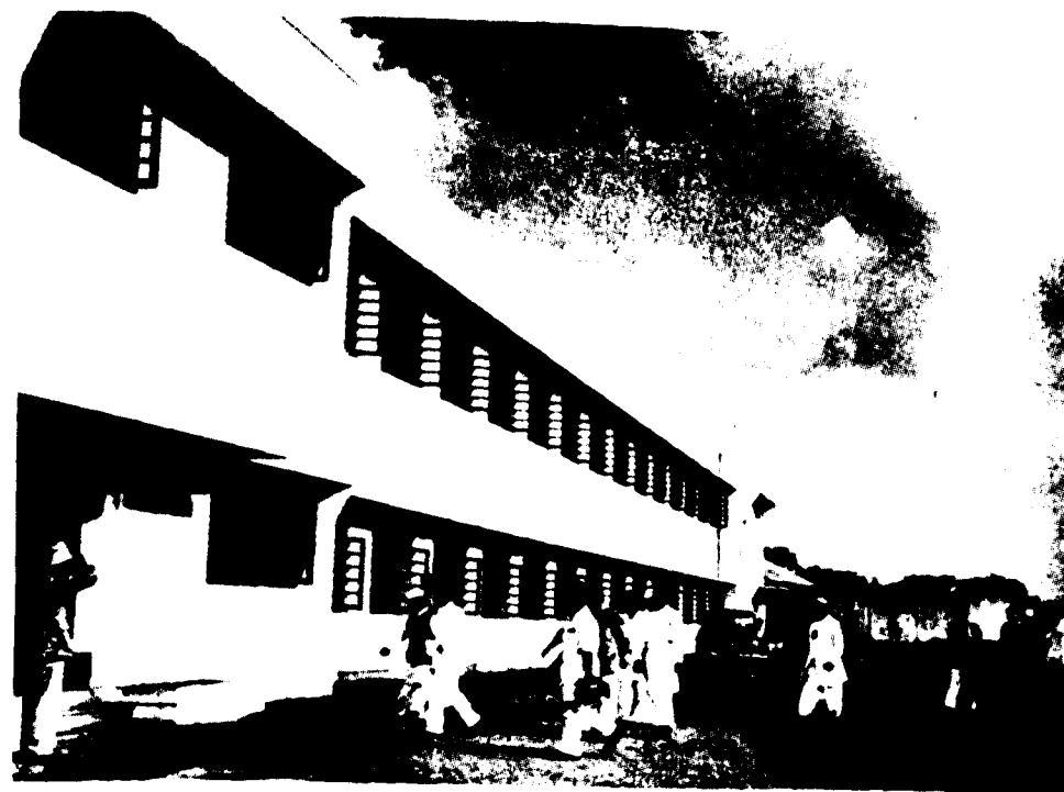
Photo shows the Canteen Building of the Integral Coach Factory.
