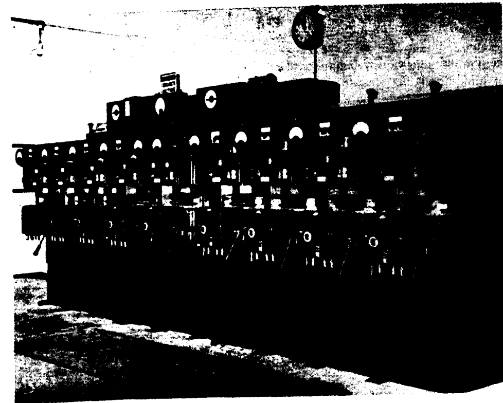
Photo shows a nine-panel 11 K. V. Switch Board at the Integral Coach Factory Receiving Station.
