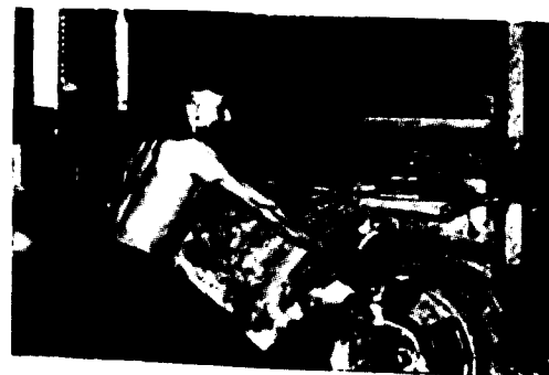
Chemicals are added to rubber in two ways. In the process shown here, chemicals are added as the masticated sheet passes between the rollers; in the other, mixing takes place in the bowels of the machine called the Banbury.
