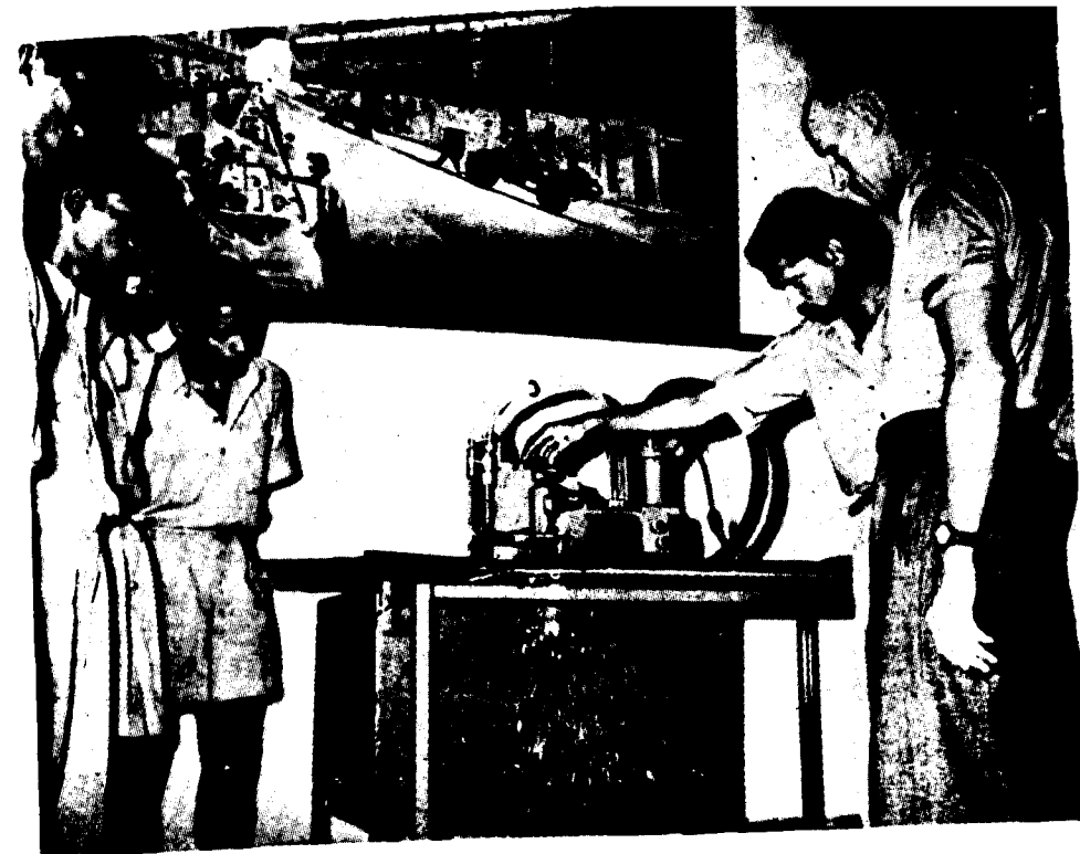
Trainees receiving instruction from a Swiss instructor in the Welding Department of the Technical Training School at I.C.F.
